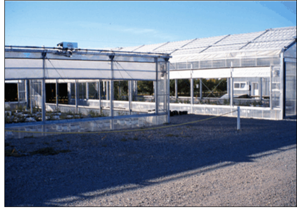
Fig. 6. A view of partially constructed and completed greenhouses – the side walls are open, the roof covering is closed. (Photo by Matt Rogoyski).
