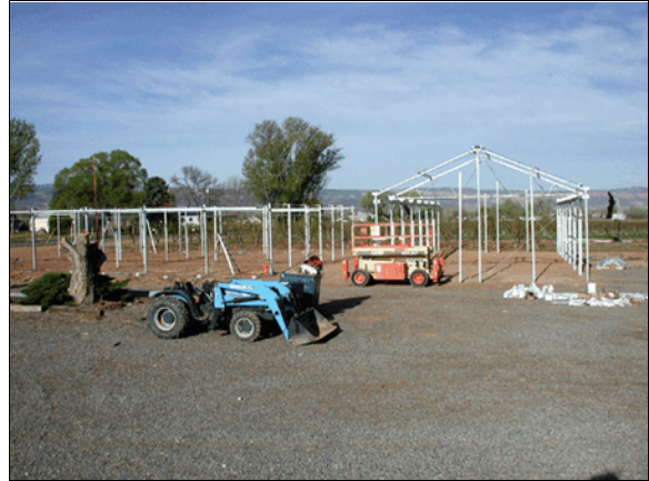
Fig. 3. Structures of the two greenhouses: the flat roof greenhouse has load bearing cables as a key structural component; trusses are the key structural component for the peak roof greenhouse. (Photo by Harold Larsen)
